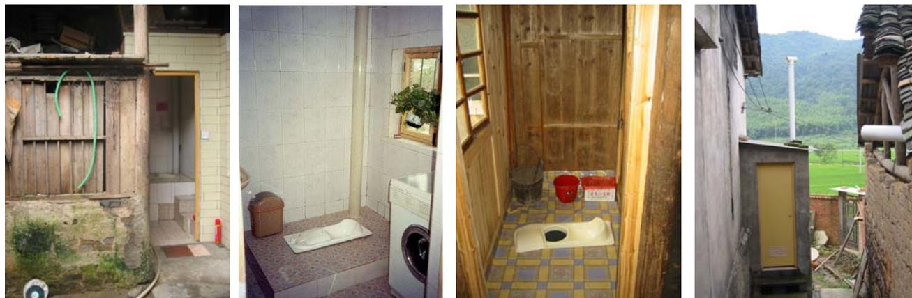
Figure 2: Different sites with urine diverting toilets: in the house yard, in-house, or outside the house (source: GTZ, Morel)
