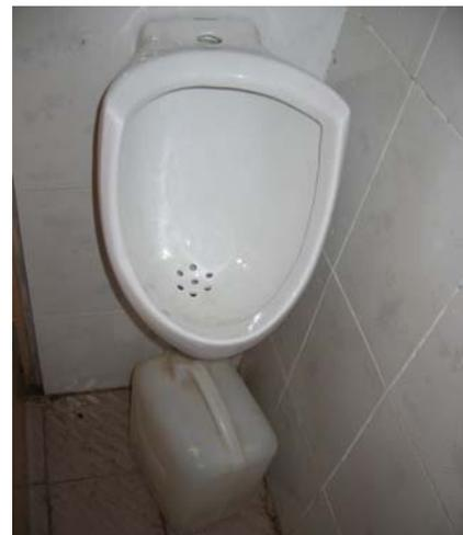
Figure 5: Urinal with canister (photo: GTZ)
