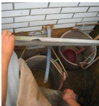
Figure 3: Urine outlet from toilet (photo: GTZ)
