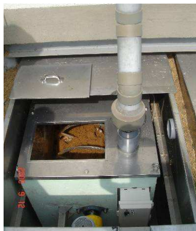
figure 4 : reactors of the permanent toilets (source: Seiwa-Denko)
