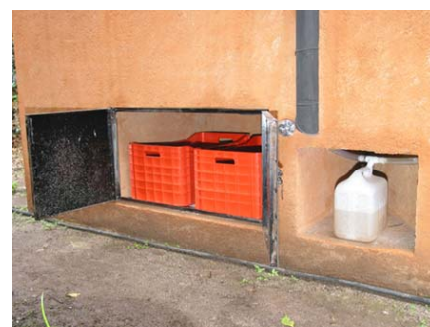
Figure 10: Dehydrating chamber with 2 containers for faeces (source: TepozEco)
