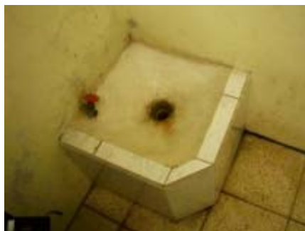
Figure 6: Urinal for women and men (photo: Xavier Zapata)
