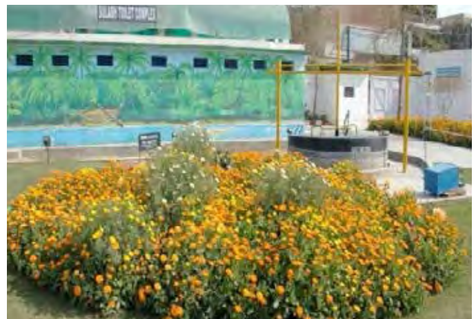
Sulabh Community Toilet linked with Biogas Plant
