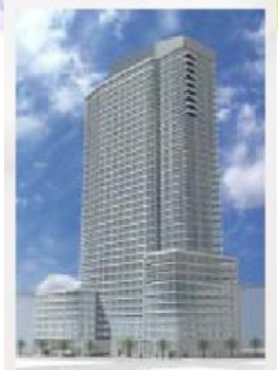
Helena Apt. Bldg, NYC (50,000 GPD blackwater to cooling water and irrigation)
