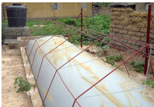
Figure 5.6 a Digester after start-up
