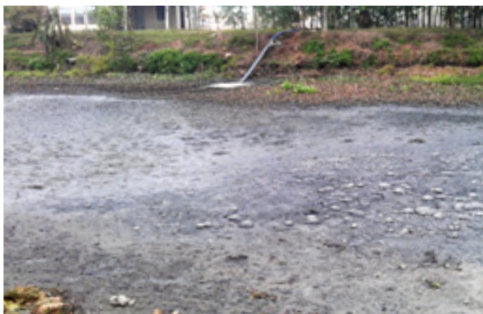
Figure 2.1 Open pond treatment system of a medium scale farm releasing methane and over-flowing into a public irrigation canal. The “before biogas” situation of Mr. Tran Van Quang’s Farm Bac Ninh province.
