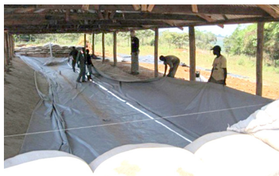
Figure 3.5 Installing the digester bag
