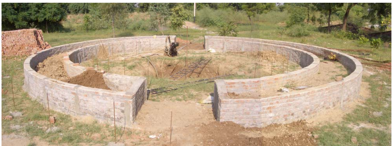
figure 8: Pic of new common sanitation complex at DSK (under construction)
