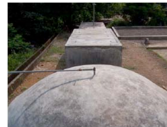
View of anaerobic treatment: digester, anaerobic baffled reactor (ABR), and anaerobic filter (AF). Gas produced from digester is piped to offal room.
