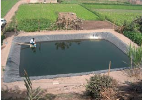
Stabilisation ponds reduce contamination risks Photo: IPES
