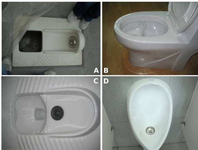
Fig. 6: Different toilet models and a waterless urinal used in the public toilet blocks. A Urine-diverting dehydration toilet (UDDT), B Urine-diverting, low flush sitting toilet, C Urine-diverting, low flush squatting pan and D Waterless urinal. (Source: B - EnviroSystems Engineering & Technology Co. Ltd., China)
