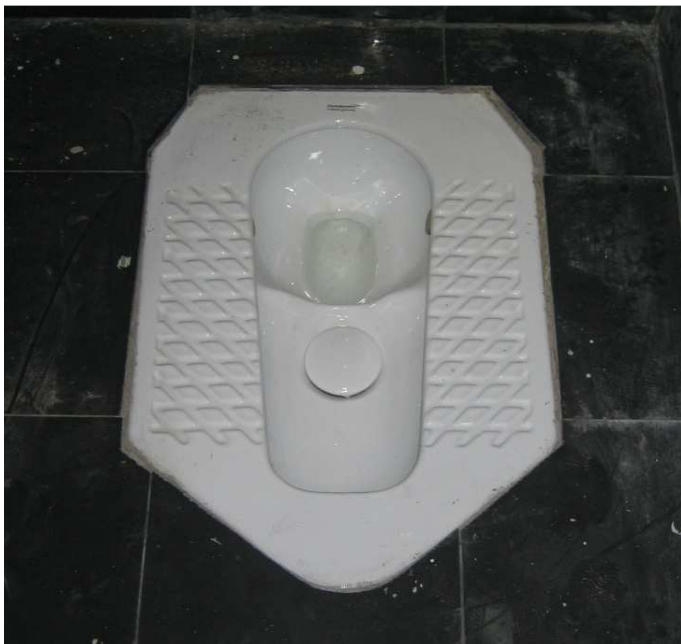
Fig. 4: Urine-diversion vacuum squatting toilet in the Sino-Italian Environment & Energy Building (source: EnviroSystems)
