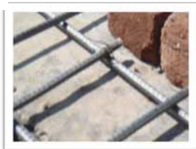
Figure 10, 11: Arrangement/Placing of Reinforcement
