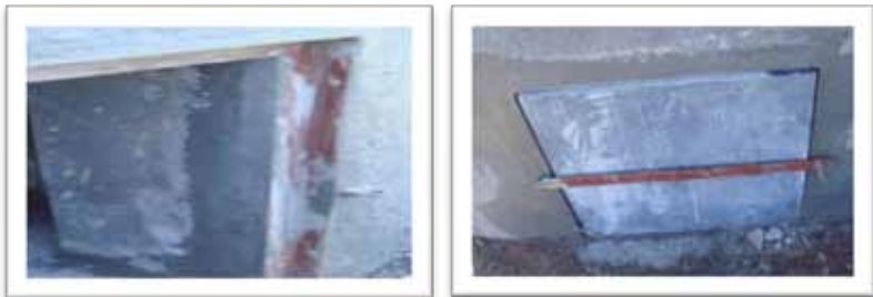
Figure 6, 7: Steel frame for the compartment opening and cover stone
