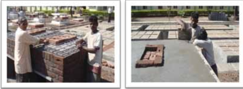
Figure 12, 13: Arrangement/Placing of Shuttering for Plinth
