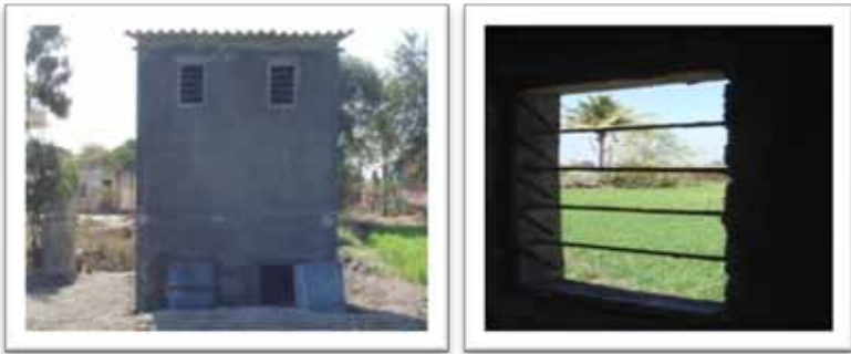
Figure 20, 21: Arrangement of Ventilator on Backside of Toilet
