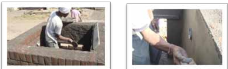
Figure 4, 5: Inside plastering of the compartment
