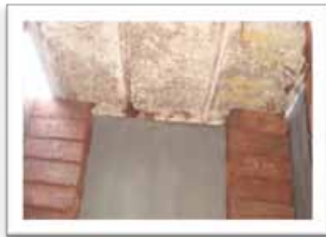
Figure 9: Supporting of a shuttering
