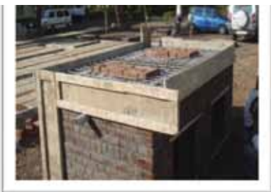
Figure 10, 11: Arrangement/Placing of Reinforcement
