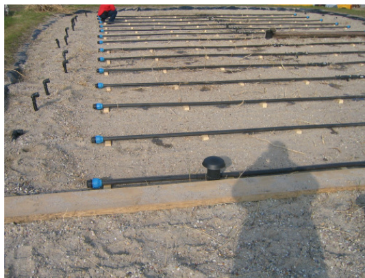
Fig. 2.4.18: Constructed wetland, distribution system
