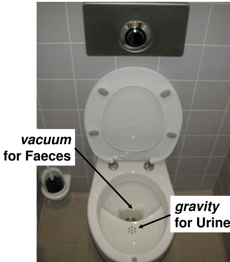
Fig. 2.4.2: Vacuum separation toilet
