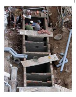
Improve existing systems: Anaerobic Baffled Reactor (ABR) as an alternative to conventional septic tanks (Hanoi, Vietnam, 2003)
