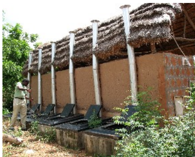
Fig 1: Ventilated pit latrines at Orphanage Africa in Ayeniah, Ghana
