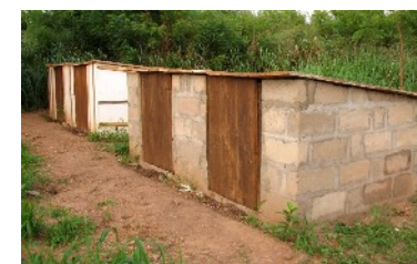
Fig 3: Permanent compost enclosures at Valley View University in Oyibi, Ghana
