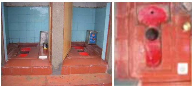
Fig. 8: Toilet cubicles (left); and top view of prefabricated urine-diversion squatting pan with washwater bowl (right) (source: seecon gmbh, August 2006)
