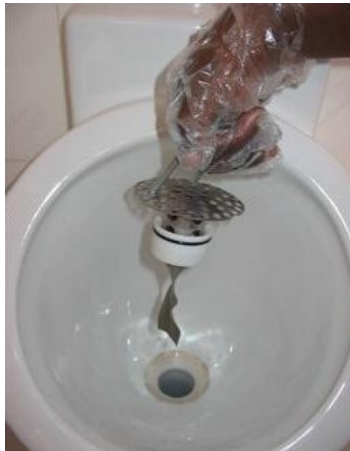
Fig 3: Membrane odour seal of a dry urinal
