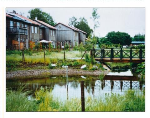
chemical precipitation, and this was why they chose a system with urine separation, a local treatment plant and subsequent treatment in ponds and ditches. This alternative was adopted despite the option of connecting up to the nearby municipal wastewater system.
