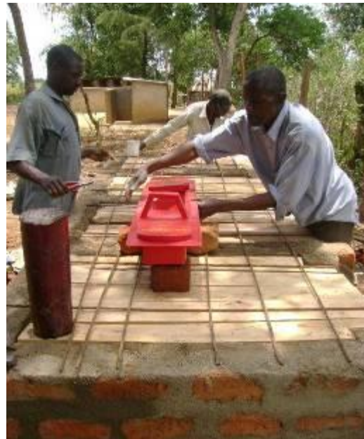
Fixing twisted iron bars, squatting pan and hole for ventilation
