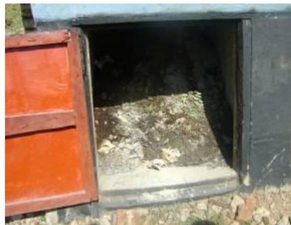
Alternative straight chamber door in Ugunja
