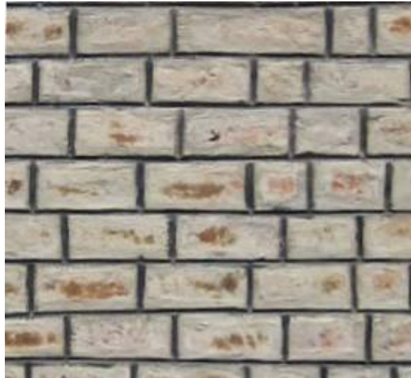
Wall surface after finishing
