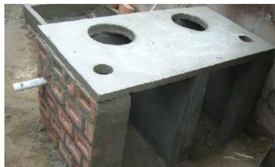
Faeces chamber and toilet slab
