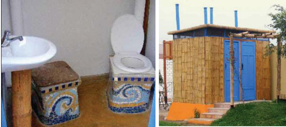
Two seater toilets and hand washing sink inside the cubicle UDDT from the outside
