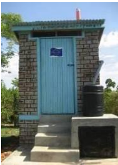
Double-vault UDDT in Ugunja (front view)
