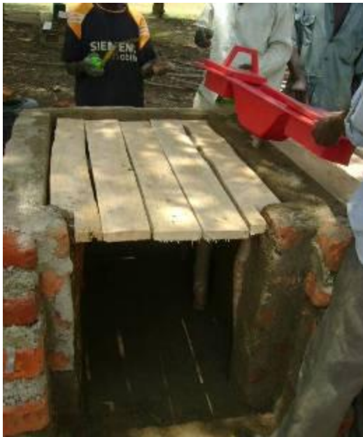
Fixing shuttering timber in the chamber wall
