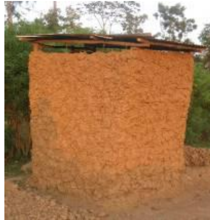
Simple local super structure from wooden sticks and earth (incl. earth plastering) in Ugunja
