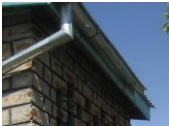
Steel gutter from the back side
