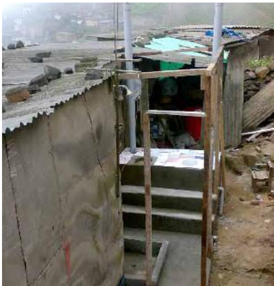
Toilet during the construction without walls
