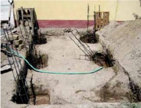
Preparation of the Ferro-cement foundation pillars
