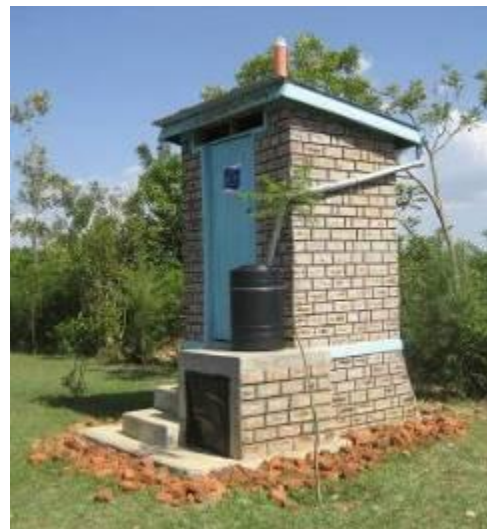
Double-vault UDDT in Ugunja (side view)
