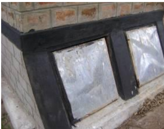
Faeces chamber doors at Rachuonyo
