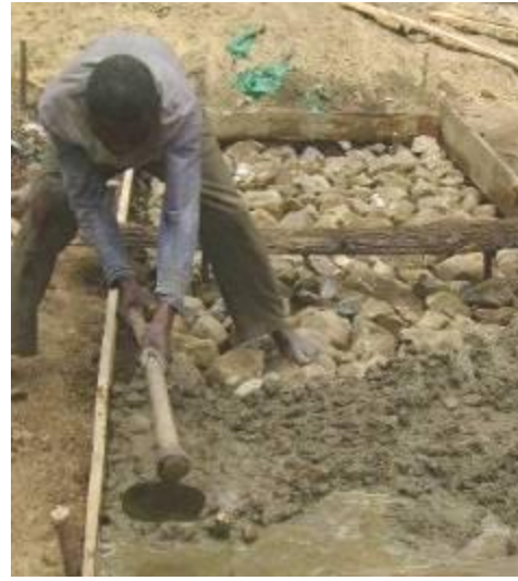
Distributing mortar on top of the ballast
