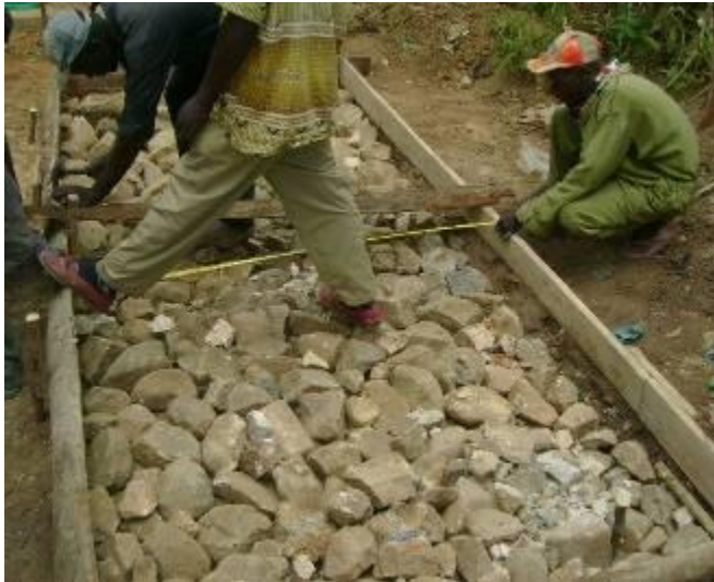
Measurement of the foundation
