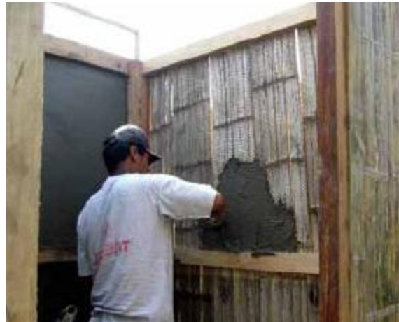
plastering from the inside of the cubicle
