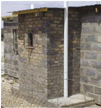
EcoSan toilet accessible from the house at a South African suburb (source: WSP, 2005)
