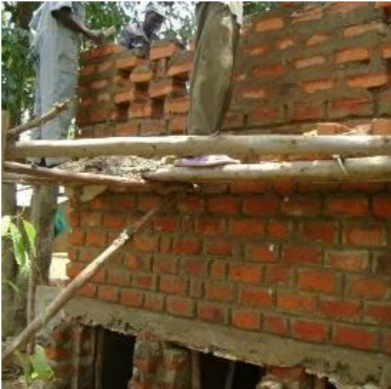
Wall during the construction
