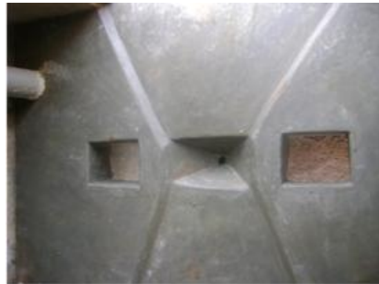
Modulated squatting pan in Kericho Unilever estate
