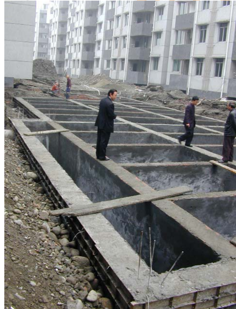
农业部能源与环境技术开发中心 Baffled septic tank ENVIRONMENTAL PROTECTION (IEEP) TECHNOLOGY DEVELOPMENT (CEEPTD/MOA)
