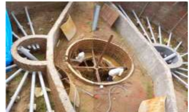
Biogas plant during construction
