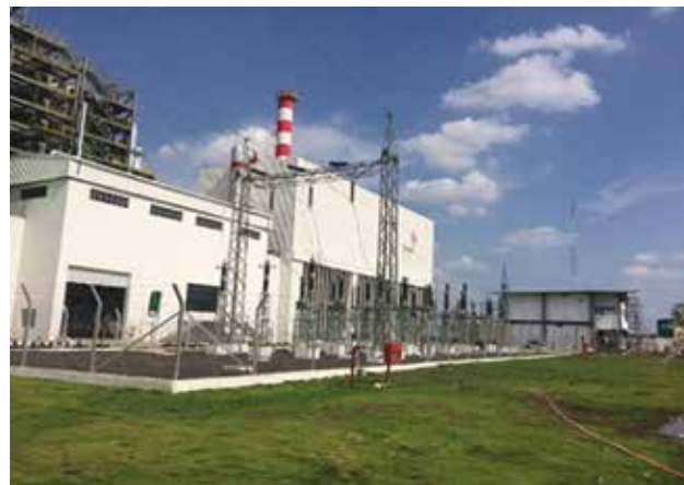
Figure 6.19: Waste-to-energy plant site in Jabalpur, Madhya Pradesh
