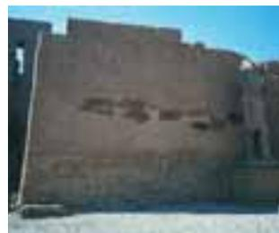
The temple of Rameses III at Karnak is damaged and discoloured (white patches) at the lower part of the temple wall. The darker patches higher up are caused by nitrate salts and indicate the ground level before the excavations; they are not associated with the present transport of groundwater up into the monument.
