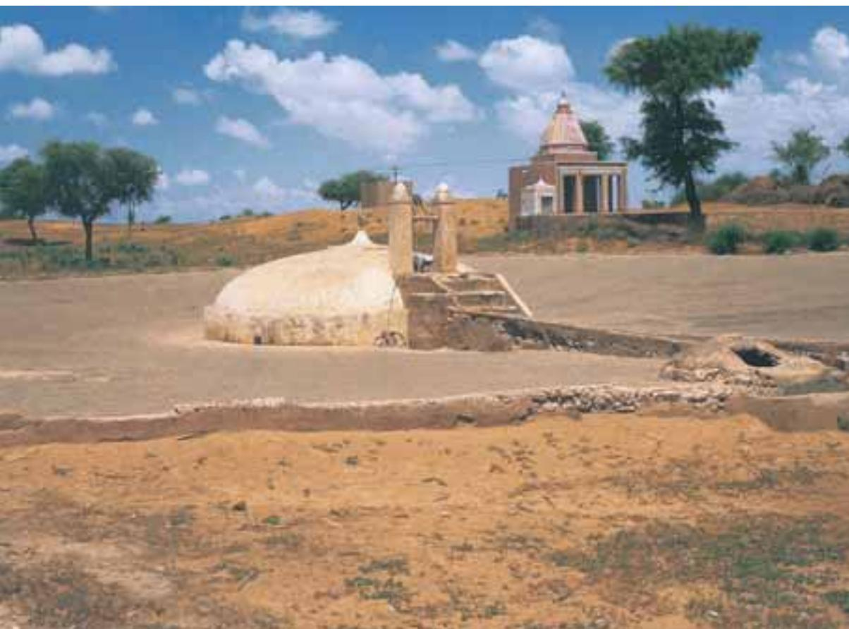
Up-end the teacup on the saucer and you have a clever way of collecting rainwater! This collection arrangement is in the desert state of Rajasthan in India. With a hectare of land and 100 mm rain, 1 million litres of rainwater can be harvested. Photograph: CSE
