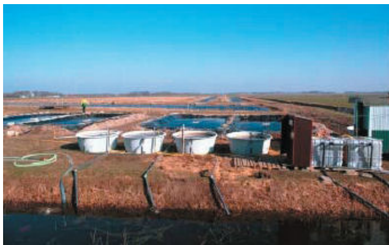
Figure 3.47: "Kwekelbaarsjes" system at STP Eversteekoo (pilot plant)
