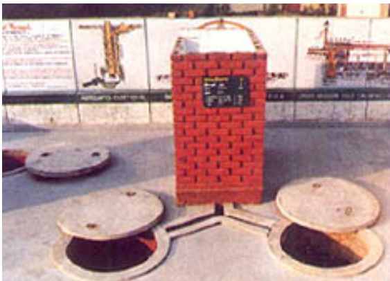
Figure 46: Two-pit pour-flush Sulabh toilet [ www.sulabhinternational.org ]
