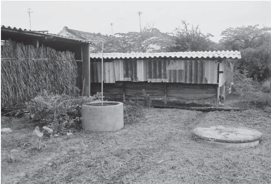
Figure 3 A completed biogas plant, only a small part of the plant is visible above ground (photo: Biogas Programme Vietnam)
