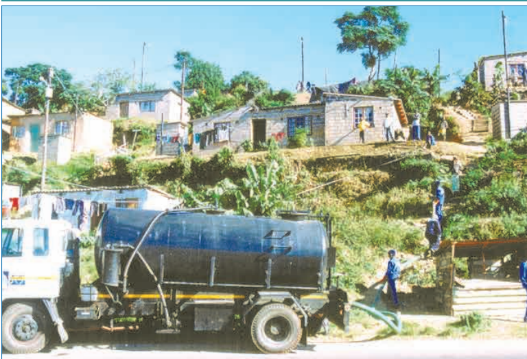
Figure 9: Problems of access by conventional desludging vehicles
