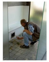
**Fig. 9:** This hatch provides access to a lever to direct urine from the urinal trough either to the sewer or to the urine storage tank (source: P. Grönwall, 2006).
