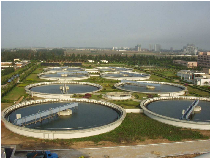
1 Wastewater treatment plant Haikou
