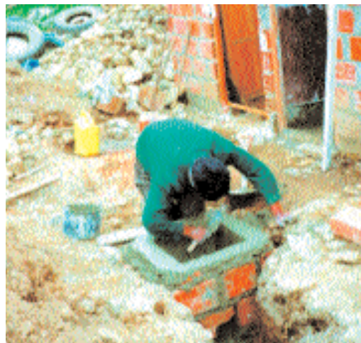
Construction of sanitary modules
