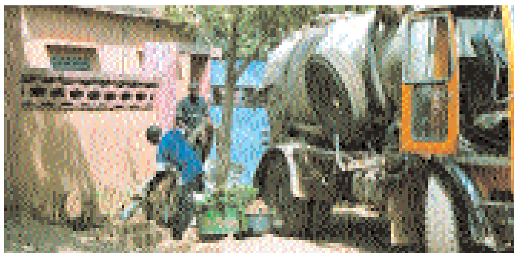
Mechanical pit emptying (West Africa)
