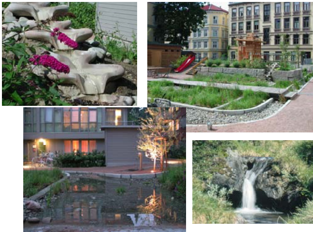
Figure 7.7. The Klosterenga greywater treatment system. Upper left; Flowforms. Upper right; the wetland in the foreground the biofilter is underneath the playground behind the stonewall. Lower left, the treated effluent is exposed in a shallow pond. Discharge to a local stream is possible as the stream was reopened. Source: Jenssen, 2005a.
