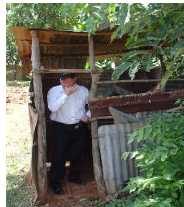
A typical pit latrine in rural households in Kenya
