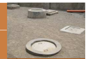
A biogas digester is located next to the facility
