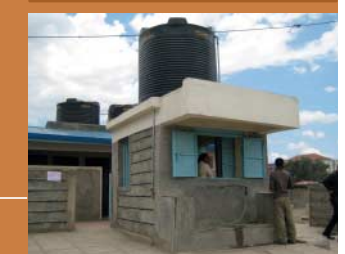
A newly built Public Sanitation Facility
