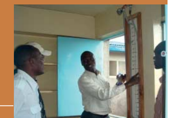
Installation of biogas appliance inside the water kiosk
