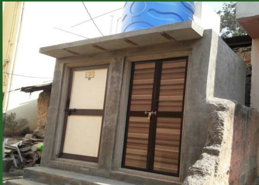
A completed group toilet in Wai.
