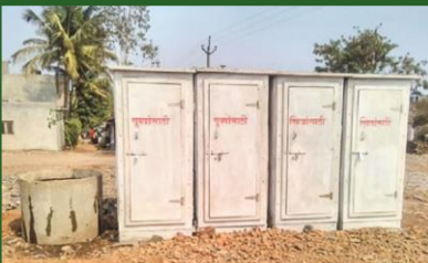
Toilets built using CSR funds.
