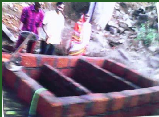
Water tanks being constructed for community toilets in Khed.
