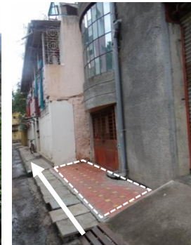
Septic tanks located near drains
