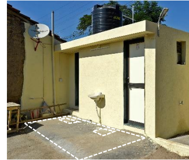
Most personal toilets connected to septic tanks
