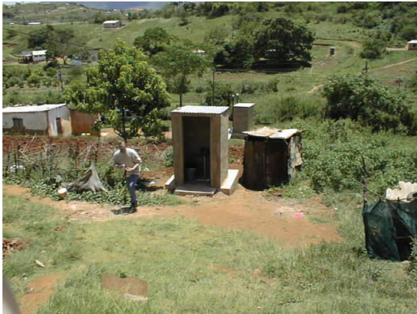
Figure 2.8: Using the natural ground slope to minimise steps at the entrance and depth of vault below ground level (Photographs: F. Stevens, eThekweni Water and Sanitation).
