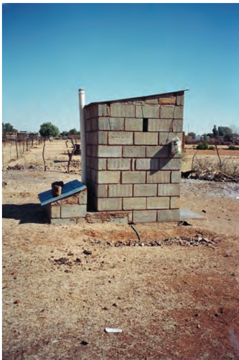
Figure 2.10: Examples of poor practice 1: It is extremely difficult to gain access to these vaults for emptying purposes (Photographs: CSIR)
