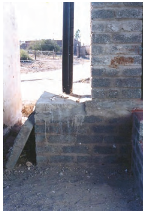
Figure 2.10: Examples of poor practice 1: It is extremely difficult to gain access to these vaults for emptying purposes (Photographs: CSIR)
