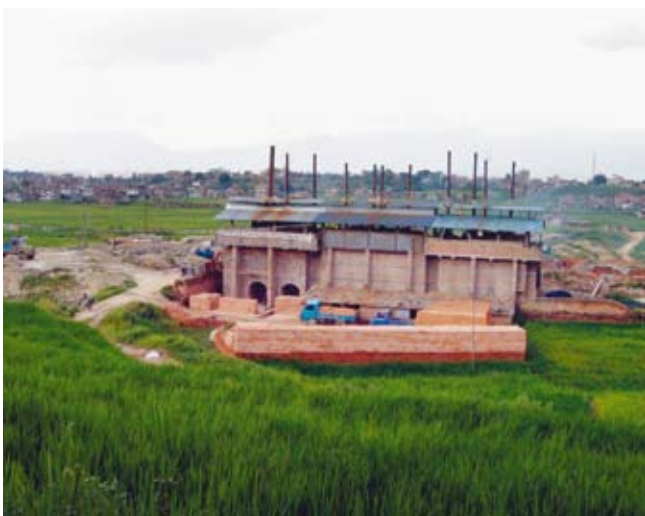
The Vertical Shaft Brick Kiln (VSBK) is the most efficient brick kiln; it saves up to 40% coal compared to conventional kilns
