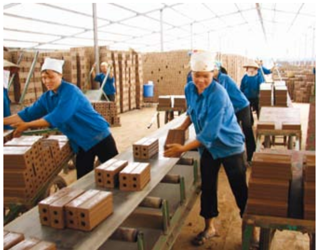
Over 300 VSBKs are already in operation in Vietnam where regulations also enforce better working conditions. Hollow bricks are popular.
