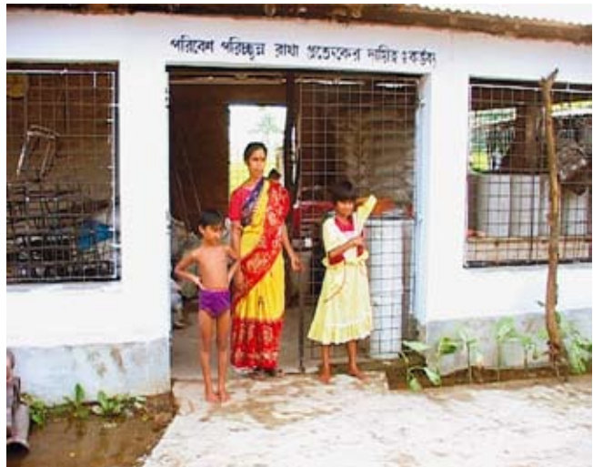
The latrines are produced by sanitation marts run by NGOs in the villages
