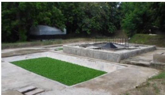
Figure 19: Ardhi University a) Photo of the system. One of the macrophyte ponds and UASB in the background. b) Schematic drawing including sampling points.
