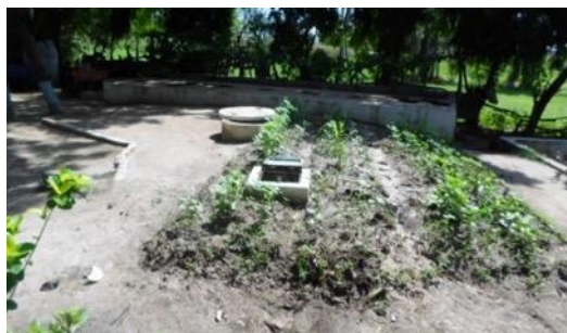
Figure 22: Kigamboni FSTP a) Photo of the system. Manholes of the BGD in the foreground and ABR/AF and sandfilter structure in the background b) Schematic drawing including sampling points.
