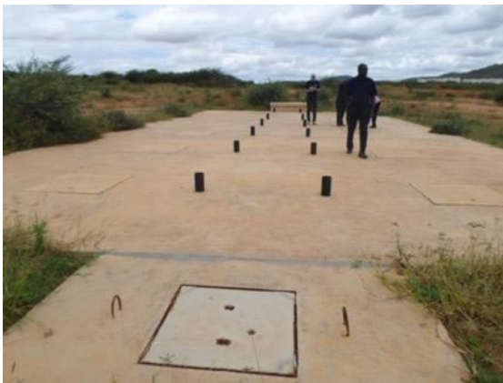
Figure 30: Dodoma University a) Photo of the system. It shows the ABR and the CW in the background. b) Schematic drawing including sampling points.
