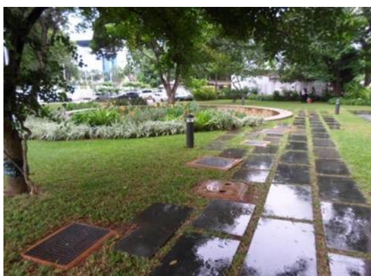
Figure 18: IST School a) Photo of the system. Manholes of the BGD in the foreground and CW in the background b) Schematic drawing including sampling points.
