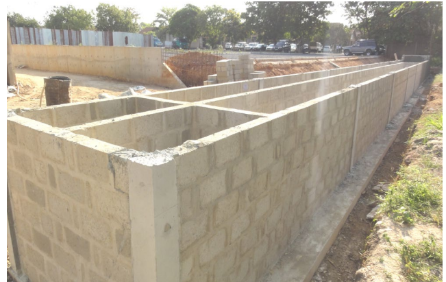
Treatment plant during construction
