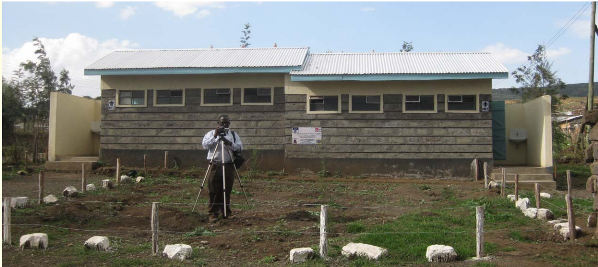
Figure 1: Sanitation facility constructed for the Crater View Secondary School.
