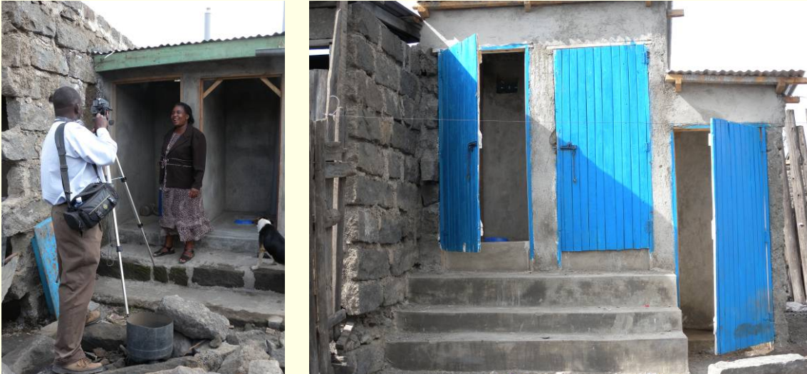
Figure 3: Two examples of privately constructed UDDTs.
