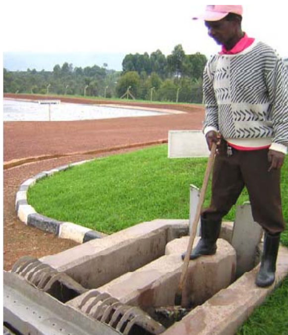
Routine works on the waste water treatment plant in Kabale
