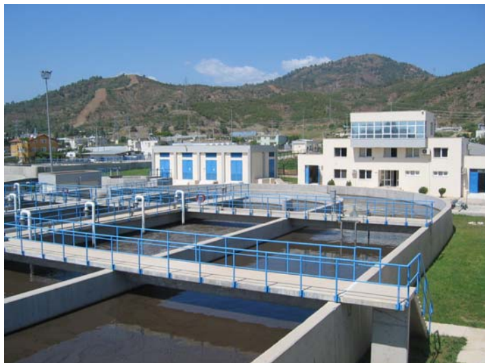
Wastewater treatment plant
