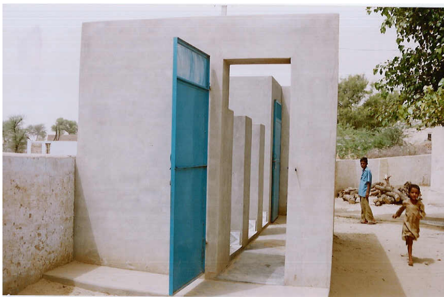
School sanitation facility
