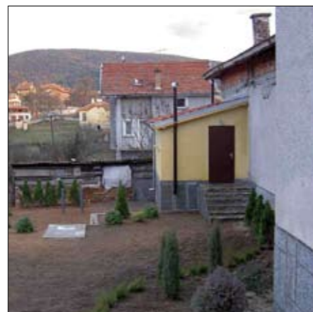
Toilet building and greywater treatment in constructed wetland
