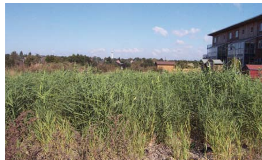
Constructed wetland for greywater treatment in Lübeck, Germany
