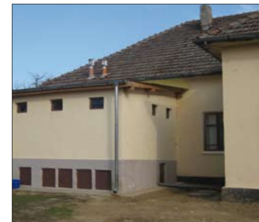
Attached toilet facility
