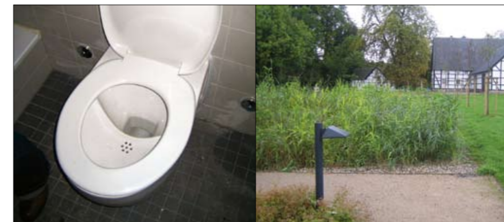
Urine diverting low flush toilet
