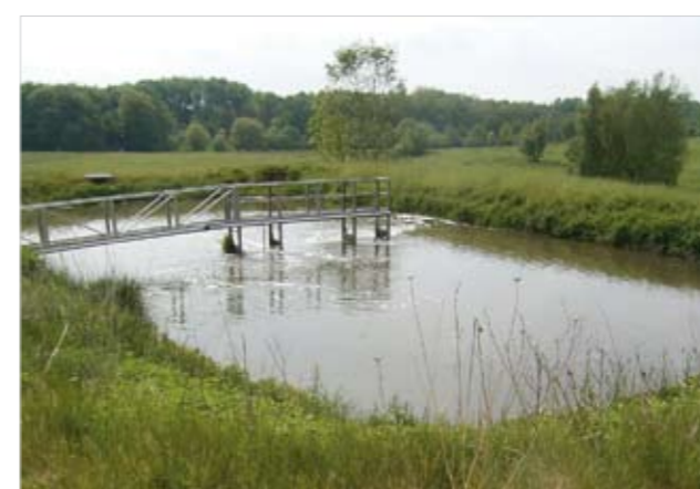
Aerated pond Schlamerdorf, Germany
