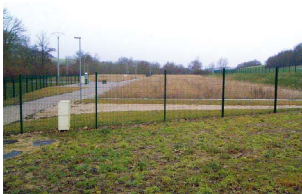
Constructed wetland without pre-treatment
