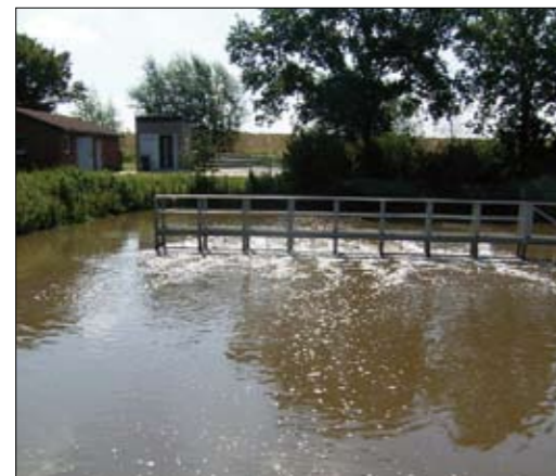
Aerated pond 1, in the background operation building (left) and building with screening unit inside
