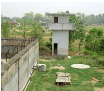
Photo 1: Biogas plant in a prison in Nepal.
