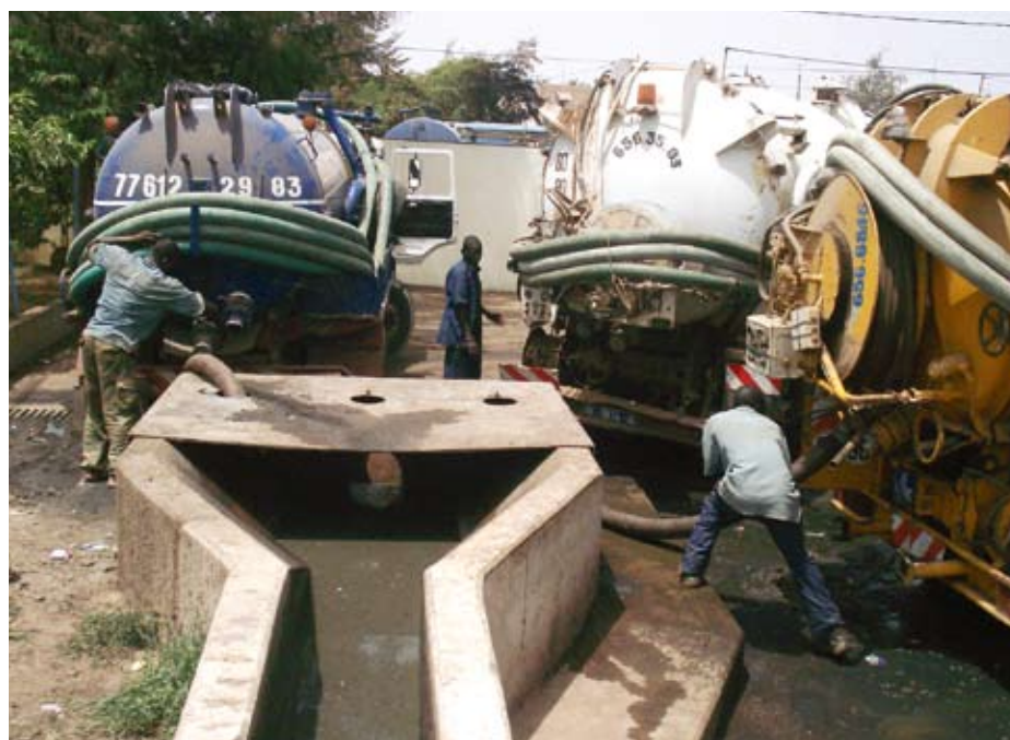
Photo 1: Faecal sludge discharge at Cambéréne treatment plant, Dakar, Senegal.
