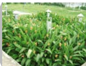
5) 2 nd Constructed wetland
