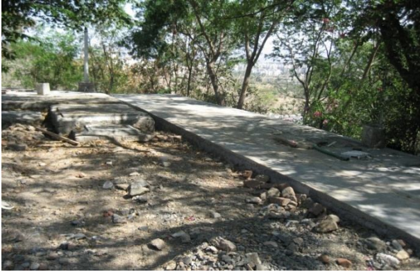
Figure 22: DTS at Oasis resort
