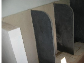
Urinals with proper gradient
