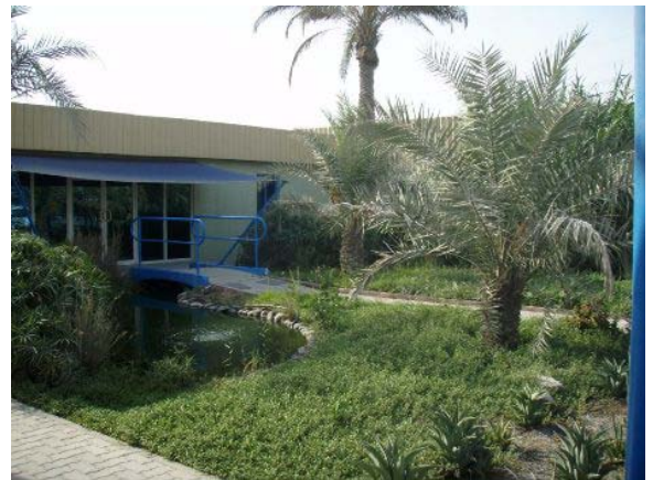
Fig. 9: Greywater garden (source: Waagner Biro Gulf)
