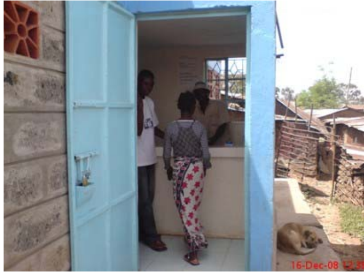
Figure 22: Silanga WC toilet
