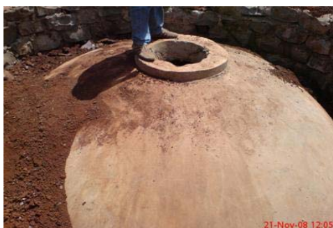
Figure 15: A bio digester (Photo taken by author)
