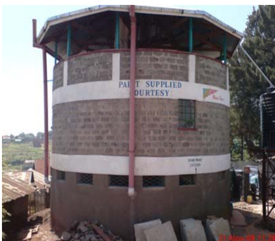
Figure 17: Gatwekera biogas toilet (Photo taken by author)
