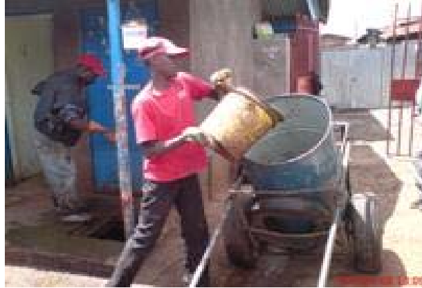
Figure 25: Scavengers emptying Line Saba VIP toilet (Photo taken by author)
