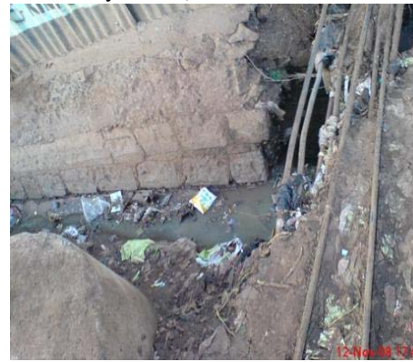
Figure 4: Hanging toilet discharging the content to the drainage channel (Photo taken by author)
