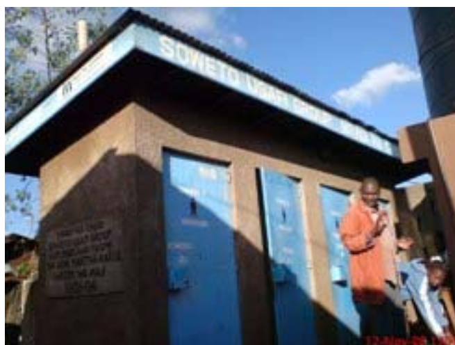
Figure 11: The selected Soweto VIP toilet (Photo by the author)
