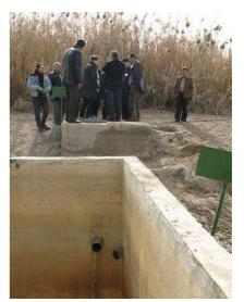
**Fig. 12:** Foreground: effluent tank with two effluent pipes discharging from the two reed beds. Background: reed beds and group of trainees (source: E v. Münch, Jan. 2009).
