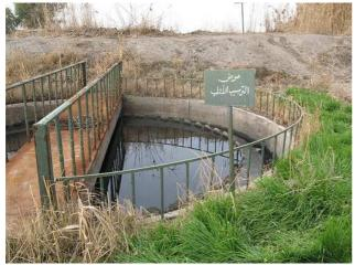
Fig: 7 Circular primary settling tank at Haran Al-Awamied treatment plant. Source: E. v. Münch, Jan. 2009.
