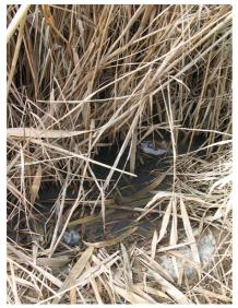
Fig. 9: Overloaded, water-logged reed bed towards outlet section of reed bed (source: E. v. Münch, Jan. 2009)
