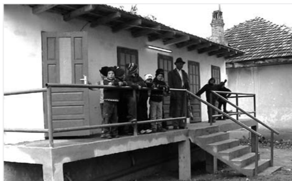
Children in front of their new toilet building. The building has 4 toilet rooms, and 1 room with 3 urinals.
